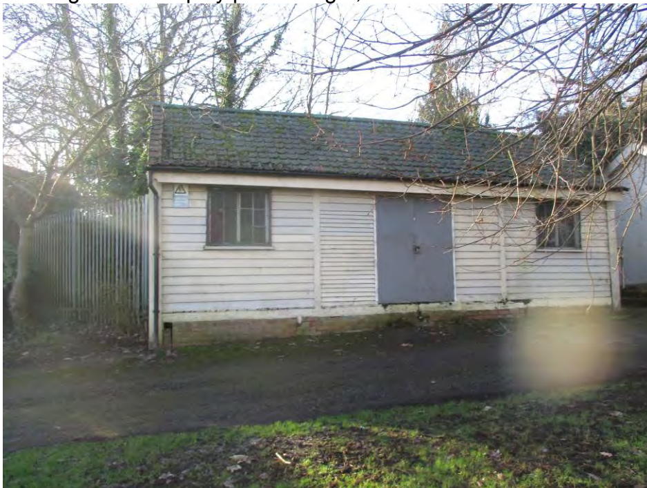
Existing structure (to be demolished)
